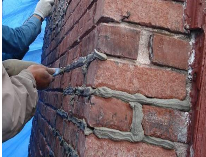
Fig1.11: Pointing wall
