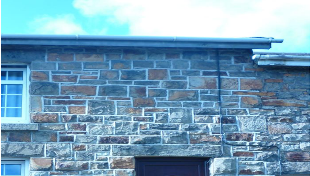
Fig1.14: Pointing surface in wall
