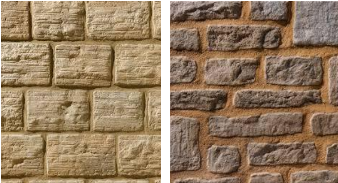
Fig.1.9 Random rubble masonry finished wall
