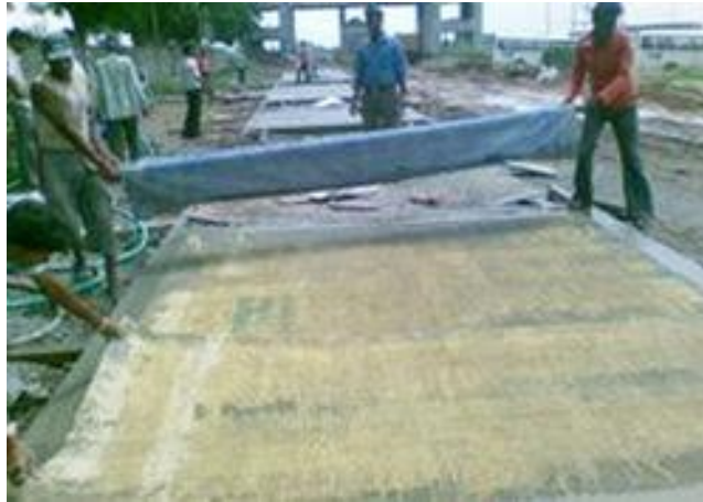
Fig 2.7 : Termix laying
