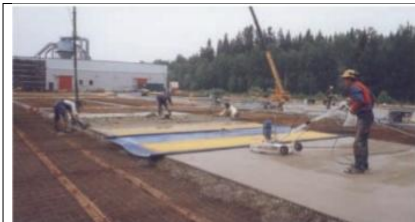
Fig.2.13: While vacuum is on, surface that has already been vacuum dewatered is floated with a power trowel fitted with a disc
