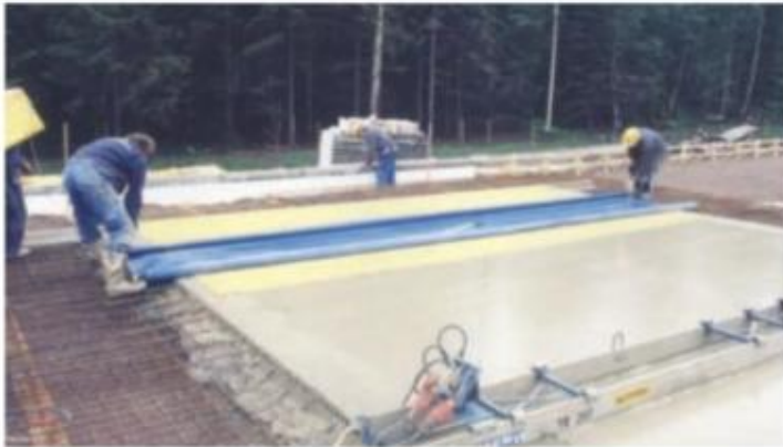
Fig. 2.11: The top cover is unrolled over the filter pads
