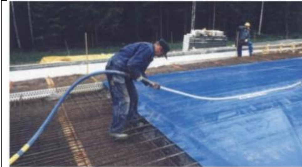
Fig.2.12 : Top cover is connected to the suction of the vacuum pump. It is important to check that top cover seals against the fresh concrete outside the filter pads
